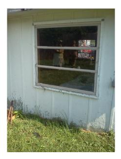
This particular window is a perfect example of a good structure upon which we could perform the "Window Takedown." We begin by taking out the window the same way we would for ventilation. Remove the glass, sashes, and frame (if made of heavy-gauge metal) along with any blinds, curtains, or window shrouds. This should be very quick work with a Halligan Bar and a Roof Hook. Once the window is gone, we move onto cutting out the area beneath the windowsill.
