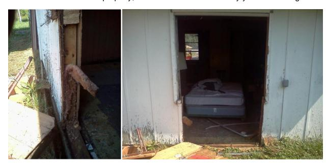
As you can see in the photo above (left), the cuts in this "Window Takedown" were made missing the jack stud, making the process an easy job. From this point we can move to accomplishing the rescue or removal. As you can see in the photo above (right), we now have created a large area giving us plenty of room to manipulate the victim out of the structure.
